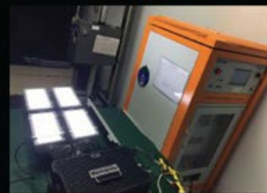
10kV prenaponski test
